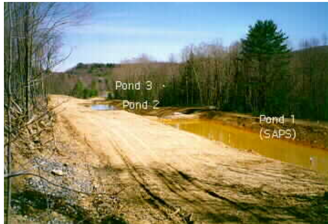
Figure 2. Overview photograph of the entire treatment system looking east from Pond 1, the vertical flow wetland (labeled SAPS here).
