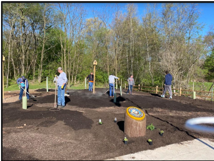
Figure 4: Pollinator garden being constructed.
