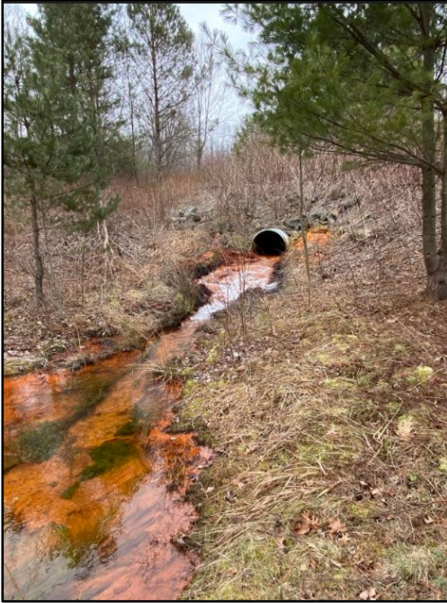
Figure 1: One of the locations on our tour with SCRA. This site is one of numerous locations where water has been directed out of the coal mines. This is one of many sources contributing to Shamokin Creek's acid mine drainage issue. No active or passive treatment is currently taking place at this site.
