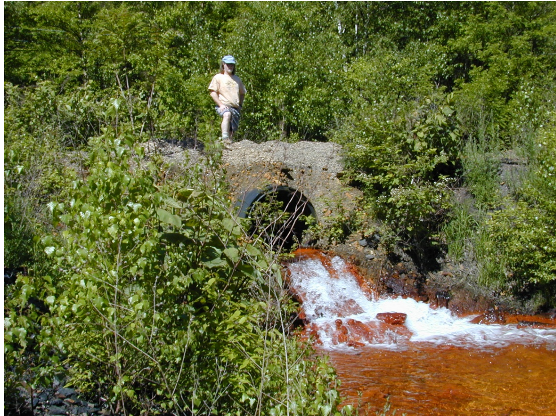
Scarlift Site 51 just upstream of Shamokin Creek near spoils pile north of Shamokin
