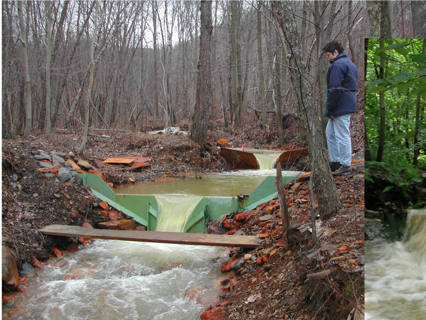
Metal V-notch weir damaged 6/27/06 flood
