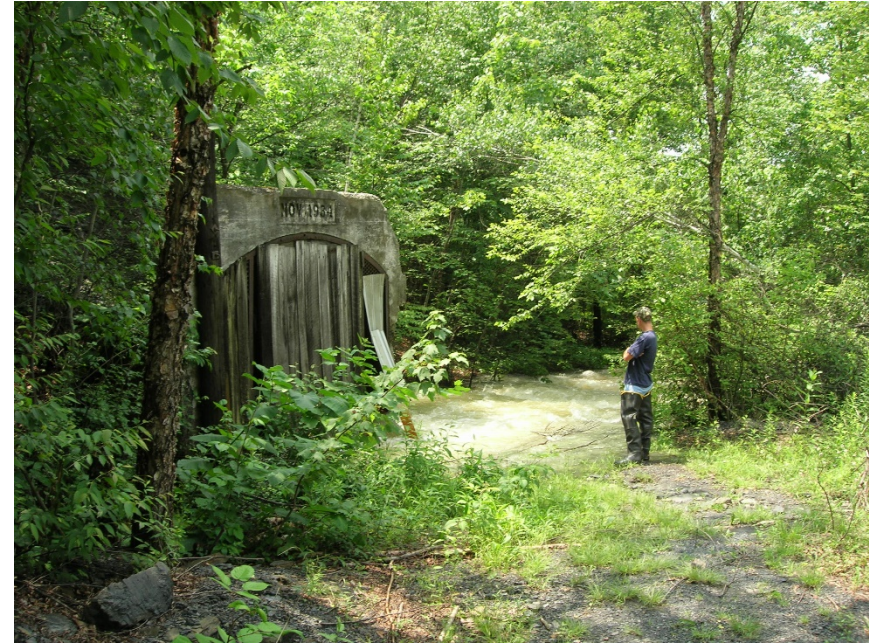
Scarlift Site 49 – pump slope
